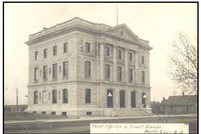
U.S. Post Office and Courthouse in Devils Lake 1910
